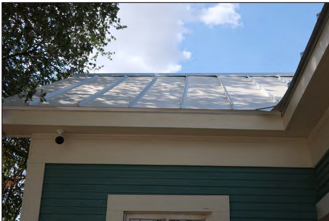
10. New Standing Seam Roof View NE
