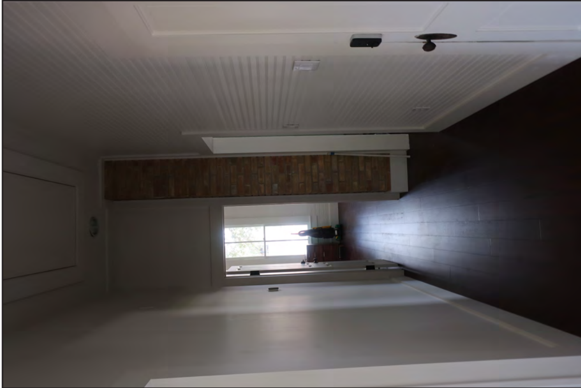
39. Hall Showing New Gypsum Board Walls, Floated Wood Floors, and Chimney View NE
