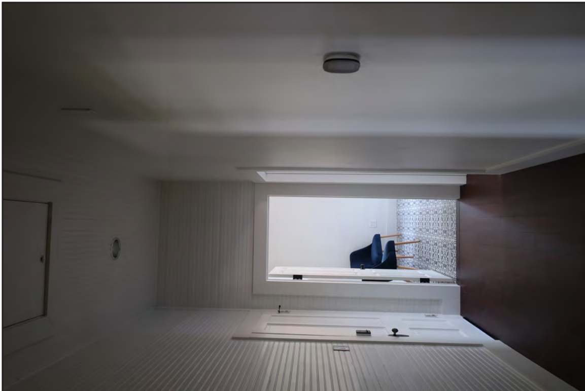
38. Hall Showing New Gypsum Board Walls and Wood Floor Installed in a "Floating" Fashion View SW
