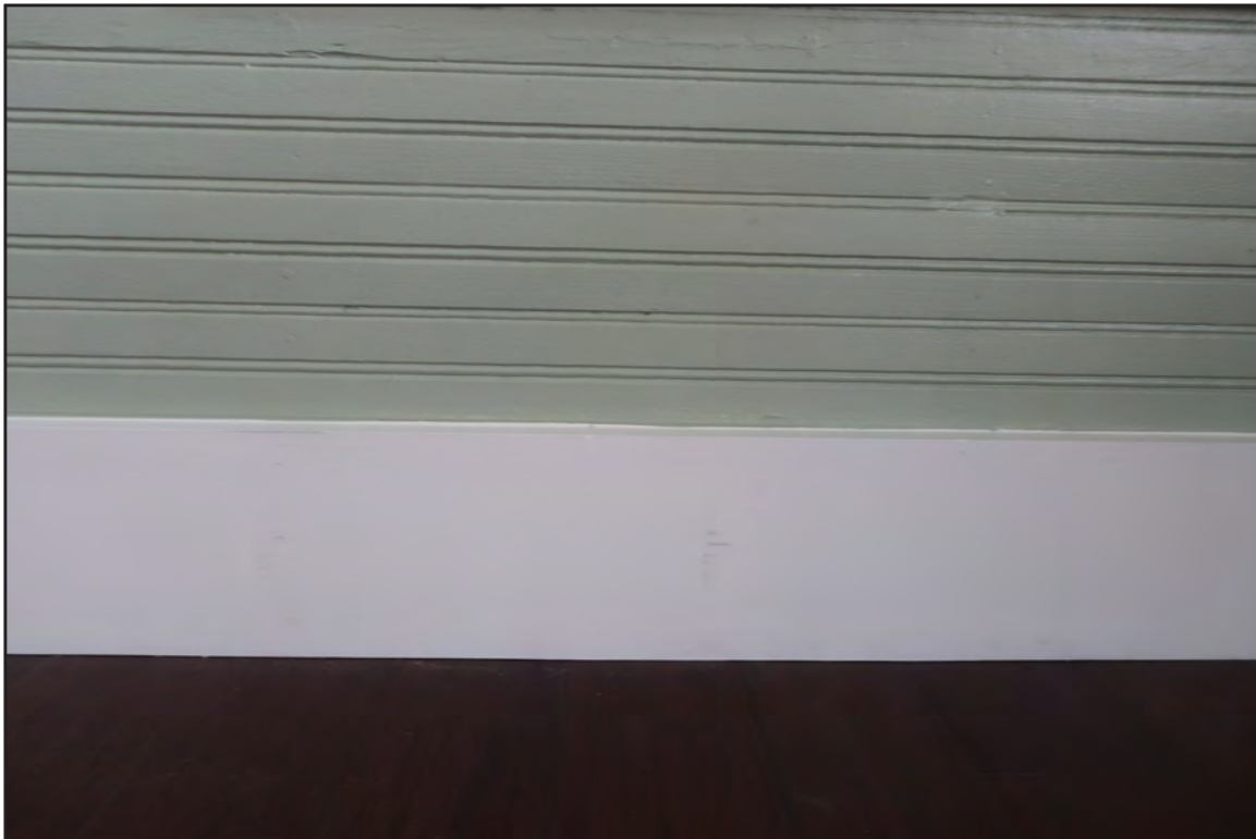
36. Restored Beadboard Walls and Trim in Reception/ Waiting Area View SE
